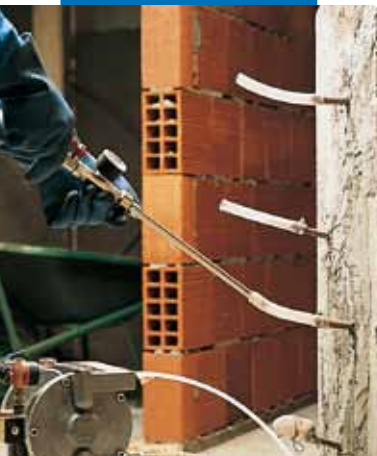
Injecting Epojet to a fissured pillar
