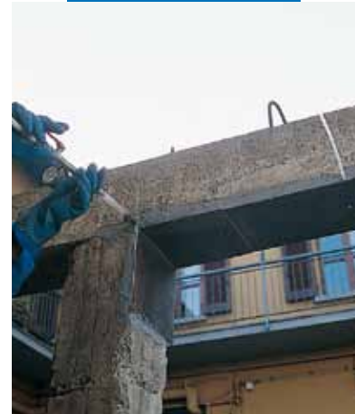
Repairing beam with injection of Epojet
