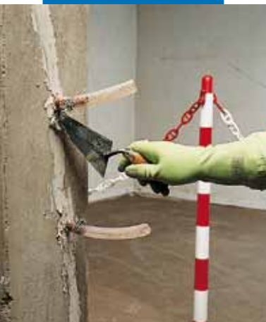
Fixing injection tubes with Adesilex PG1
