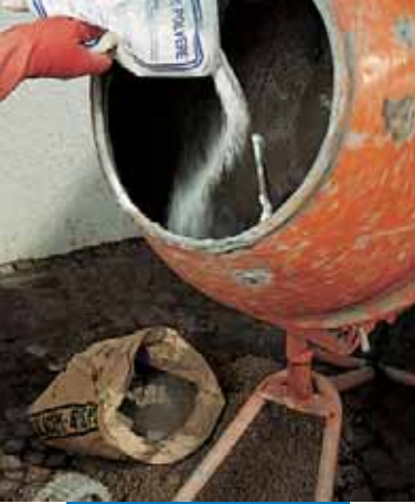
Preparing waterproof mortar admixed with Idrosilex Powder
