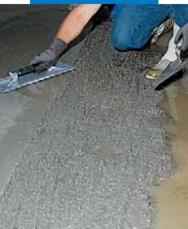
Screeding with mortar admixed with Idrosilex Liquid
