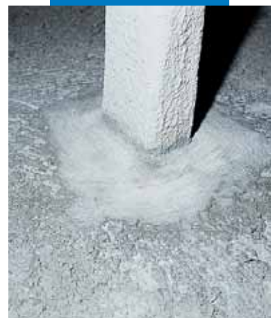
Column waterproofed with Idrosilex
