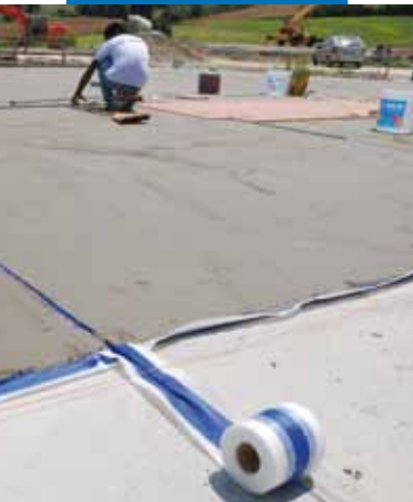
Waterproofing screeds with Mapelastic and Mapeband
