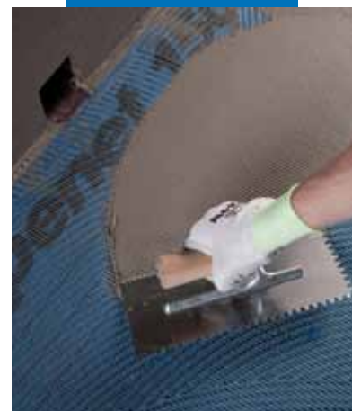
Laying Mapelastic on Mapeket 150
