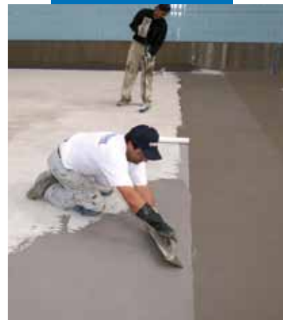
Waterproofing a swimming pool with Mapelastic
