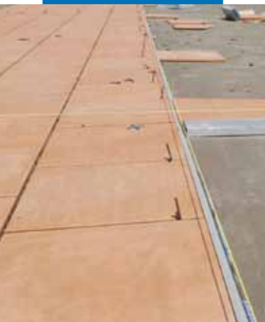
Installing ceramic with Kerabond + Isolastic
