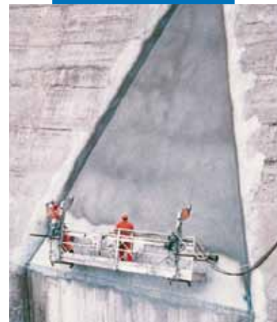
Example of Mapelast applied on a dam by spraying
