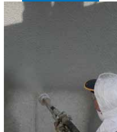
Example of Mapelast applied on a viaduct by spraying
