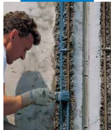
Application of Mapefer
