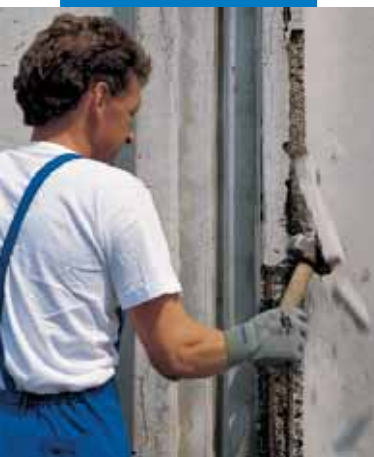
Demolition of degraded concrete
