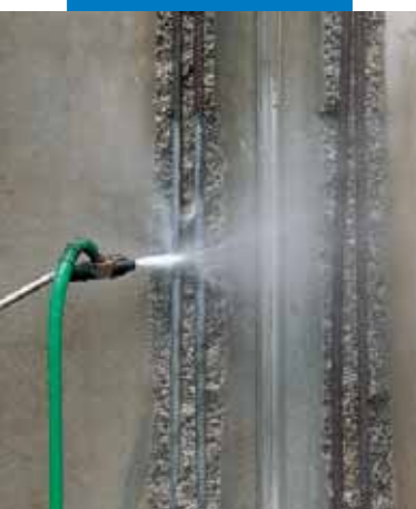
Cleaning reinforcing rods
