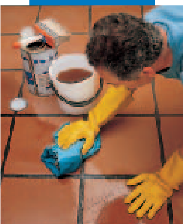
Spreading with a cloth
