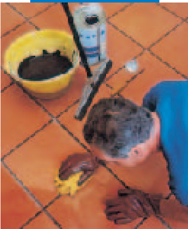
Treating cotto toscano before grouting
