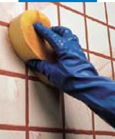
finishing wall with a sponge (still fresh grout)
