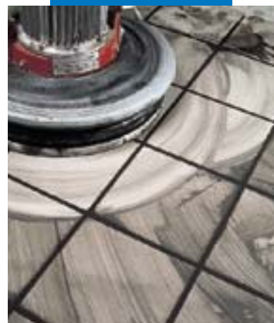
Floor finishing with a disc-type power float
