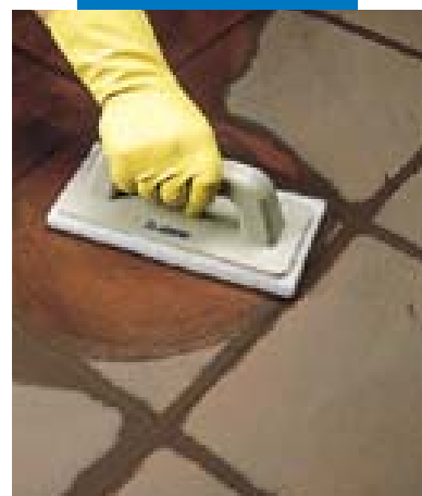
Finishing terracotta floor with a Scotch-Brite® pad
