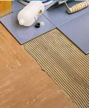
Laying on an old PVC floor
